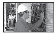
For every circuit you move to the transfer switch, connect the white neutral wire to the neutral bar in the distribution panel.
